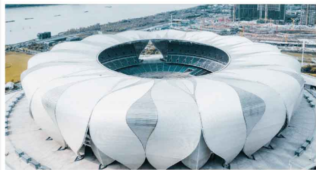
Hangzhou Olympic Center Project
