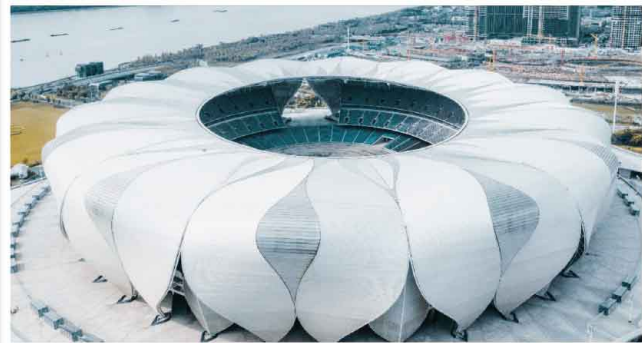
Hangzhou Olympic Center Project
